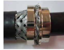
Marked 'X' for wire braid armour ring (3)
